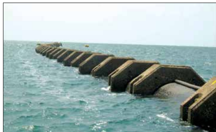
Photo 1. PE Pipe 1600 mm, Seawater intake pipe at Chennai, Desalination plant.
