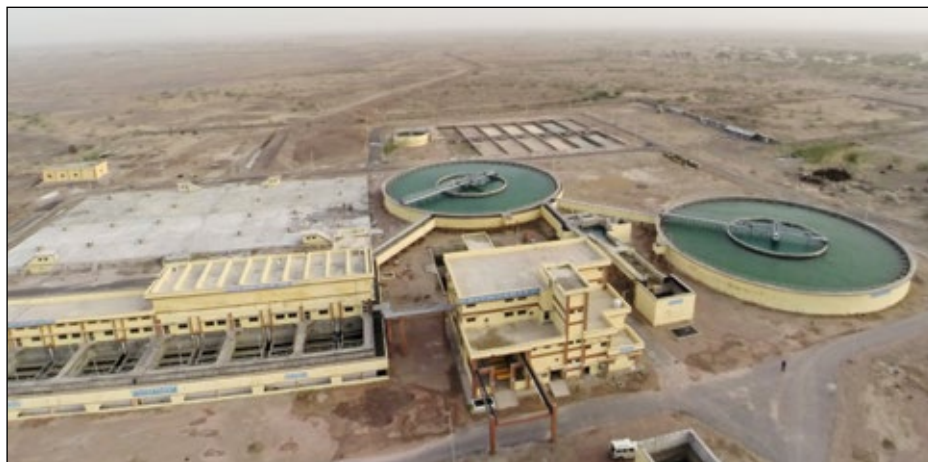
Aerial View of Pokhran Water Supply Project
