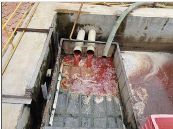
Raw wastewater from slaughter-house
