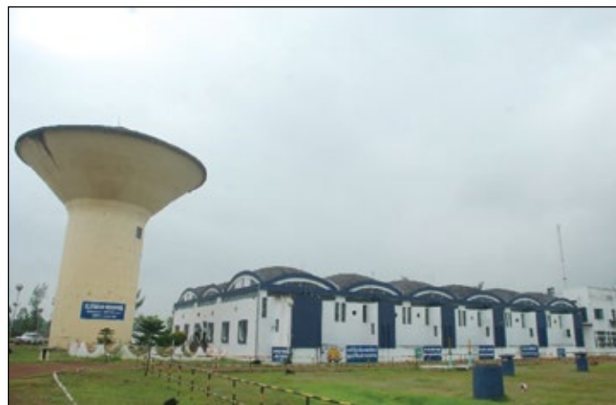
OLD WATER TREATMENT PLANT
