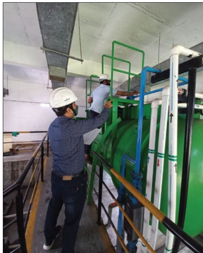
Plant audit at a Thermax customer site
