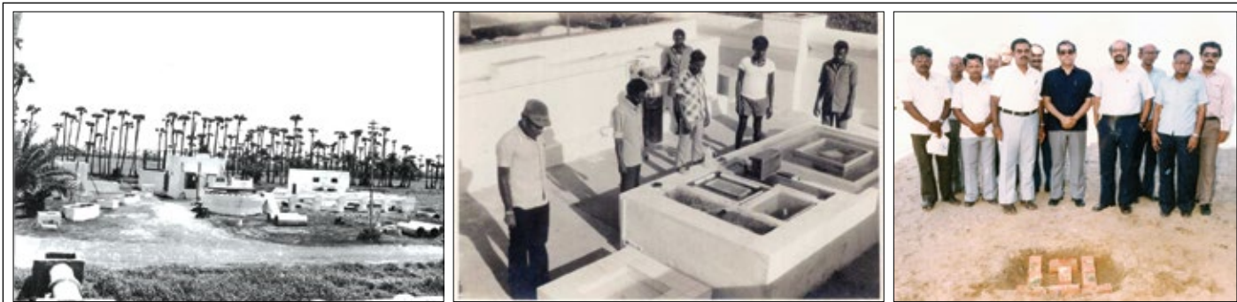
Fig. 2. The early R&D Pilot Plants of 1965 at Chennai to study Kinetics in Activated Sludge, Trickling Filter, High Lime, Carbonation 1 and 2 stages and the ground breaking of Prototype in 1988 in MFL
