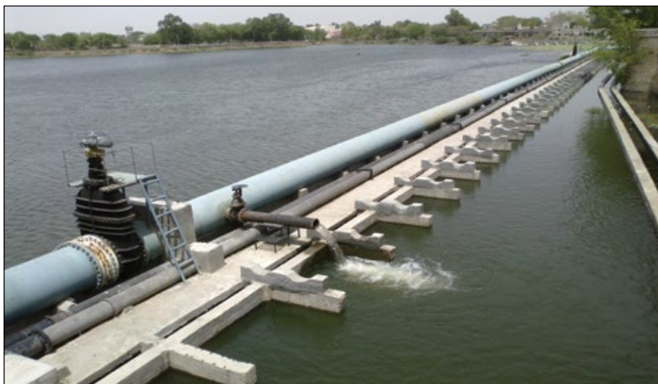
Water Supply Pipeline, Pali, Rajasthan
