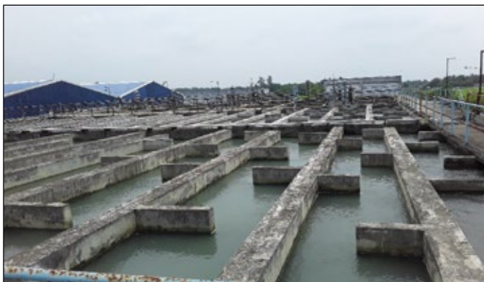
NEW WATER TREATMENT PLANT
