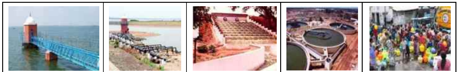
Fig.5. Chennai Water Supply in monsoon failures. Pumped water, cascade aerator, WTP and Tanker supply
