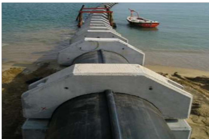
Marine Applications: (Bay of Bengal) PE Pipes installation in sea water intake for desalination plant at Chennai Municipal corporation. Himalayas region for drinking water and waste water transport.
