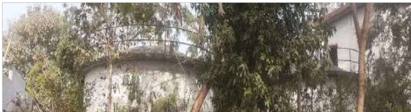
Fig No. 7 Reservoir
