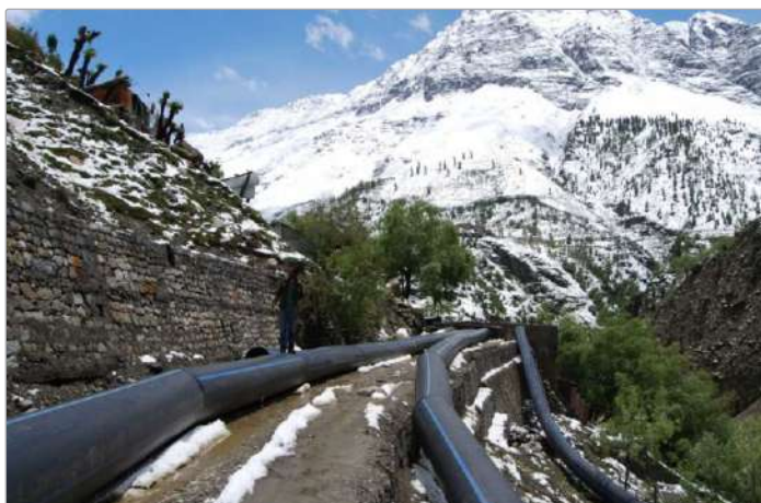
Application in Cold Climate & Hilly Terrain PE pipes resist water freezing sub-zero temperatures at 14,000 ft altitude. Himalayas region for drinking water and waste water transport.
