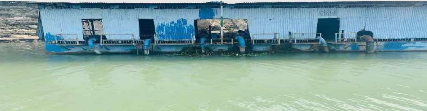
Fig No. 5 Existing Pump Barge
