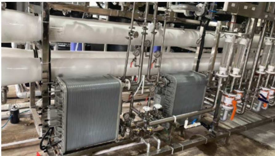
Our installation at the site
