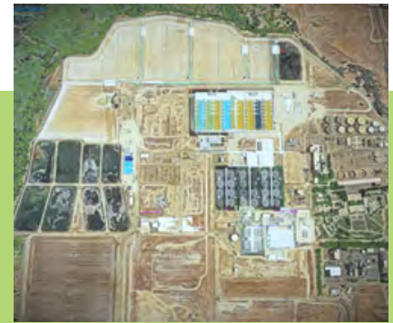
Caption: EchoWater project Courtesy of: Project Controls Cubed LLC
