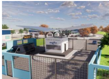
Amagua’s project involved designing a self-sustainable, energy-efficient plant, using all solar panels to power the pumps.
