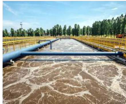
Wastewater Treatment Facility
