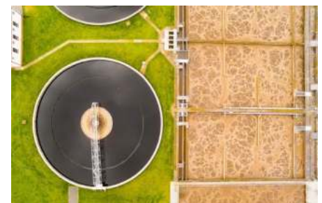
Wastewater Treatment Plant
